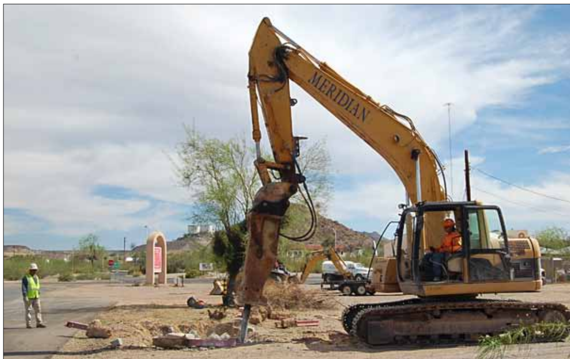
There was a big piece of equipment hard at work last week as Meridian Construction deployed this jackhammer to remove an abandoned meter box behind the warehouse of the former Phelps Dodge company store. Photo courtesy Lito Castillo
