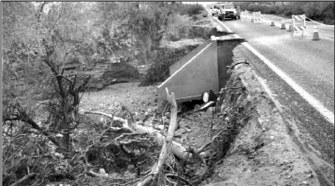
Raging storm water could not pass through this concrete box culvert beneath Highway 85 fast enough and gouged out a substantial chunk of real estate around it during recent storms at Organ Pipe Cactus National Monument. ADOT and Organ Pipe crews worked for two days repairing the road edge before both lanes of traffic were opened again. Organ Pipe photo
