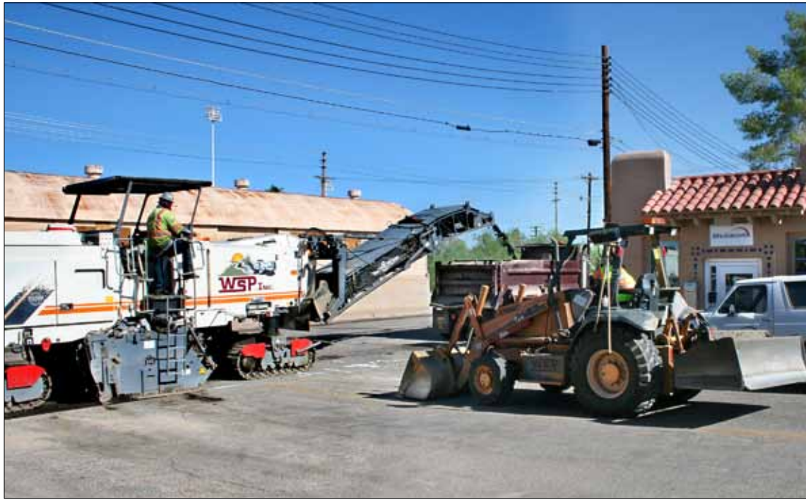
Road resurfacing has begun in some parts of town served by Ajo Improvement Company. Contractor-operated heavy equipment grinds off a top layer of asphalt and sends it via conveyor belt to a leading dump truck while street-sweepers and other equipment bring up the rear in a well-orchestrated demonstration of teamwork.
