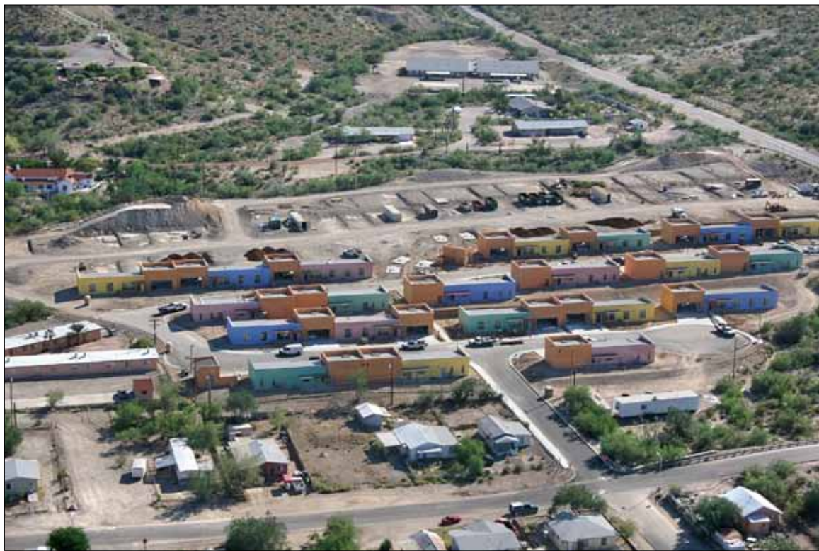
This is a recent aerial shot of the 55 Sahuaro housing complex under construction at Esperanza and Sahuaro, submitted by Robin Coachman, Housing/Project Manager with US Customs & Border Protection. While the exterior colors have raised some eyebrows, color design was based on existing colors found in Ajo structures, according to project personnel.
