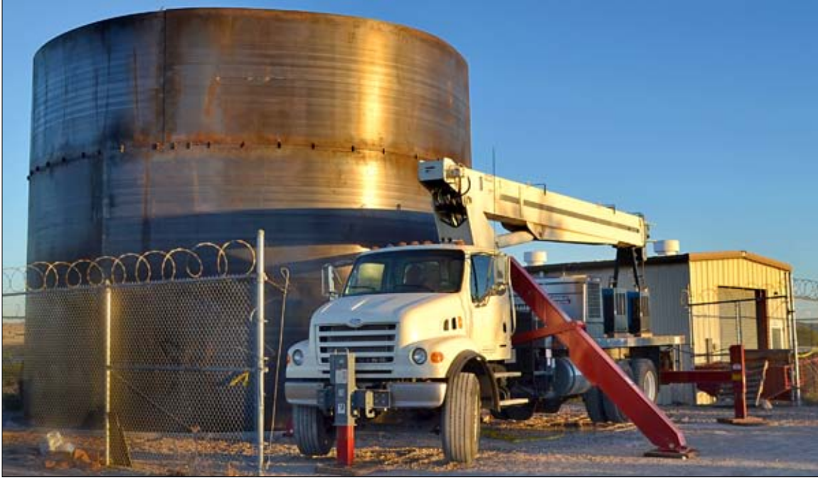
Installation of the replacement water tank serving the Ajo Domestic Water Improvement District, formerly known as the Five Acres Water Company, should be completed in the next two weeks, according to Doyle Ivey. The 125,000-gallon, 26-foot-tall tank will serve between 140 and 150 residences when up and running.
