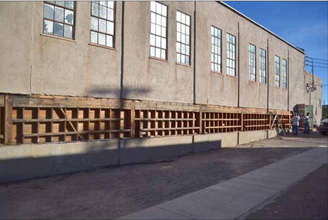
The west wall inner structure of the old Curley School gym has been opened up as part of a maintenance project being undertaken by Pima County. Once water damage has been repaired, the exterior finish will be replaced and repainted.
